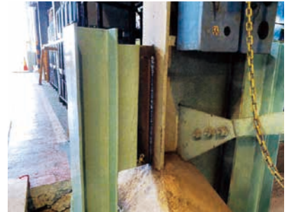
3 補強柱設置・溶接作業
